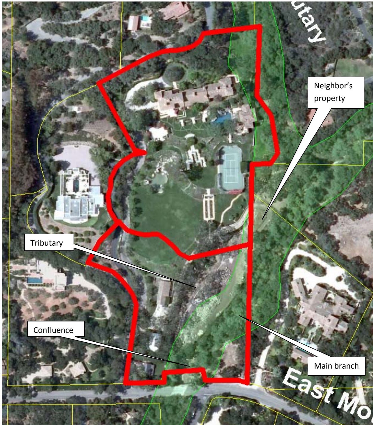
2008 Aerial Photo of Bagdasarian Property – Work is apparently underway on the peninsula between the creek channels. Construction and stockpiles of rock are visible. Notice construction on the neighbors' property to the east and apparent tree removal. Refer to Attachment I for more recent photos from the ground.
