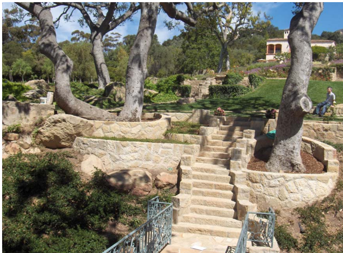
August 5, 2009 – At north bridge, new retaining walls, tree wells around oaks.
