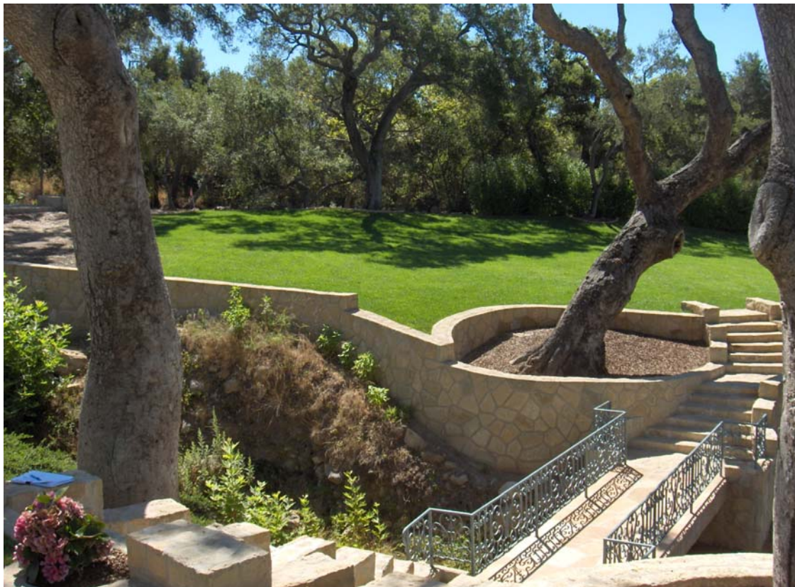
August 5, 2009 – North bridge over tributary, retaining wall, tree well around oak. Note the sycamores re-sprouting in creek.
