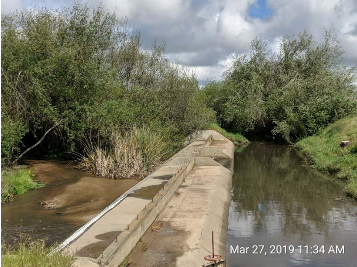
Santa Maria Airport Ditch - Section 4
