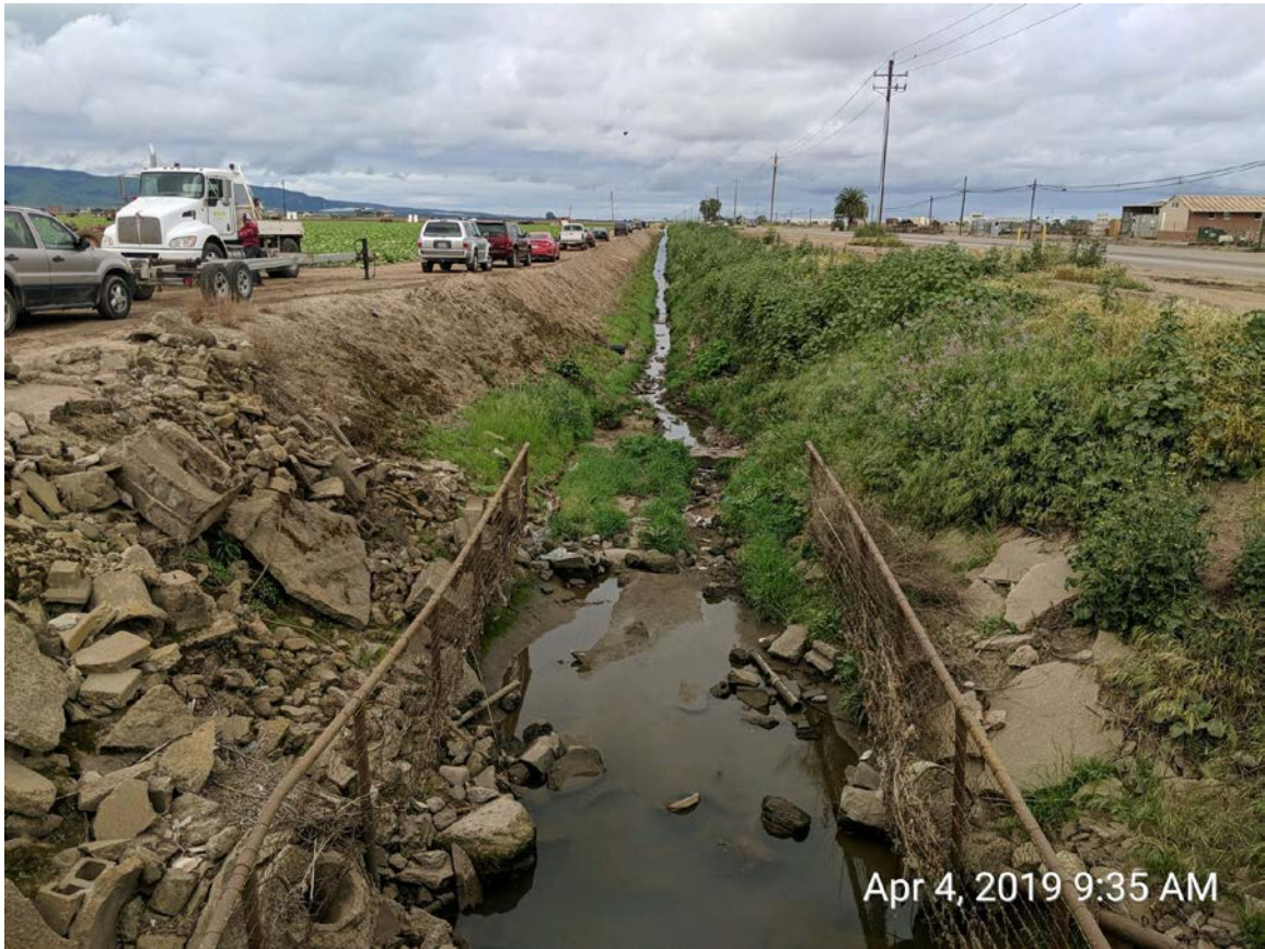
West Main Street Ditch - Section 2
