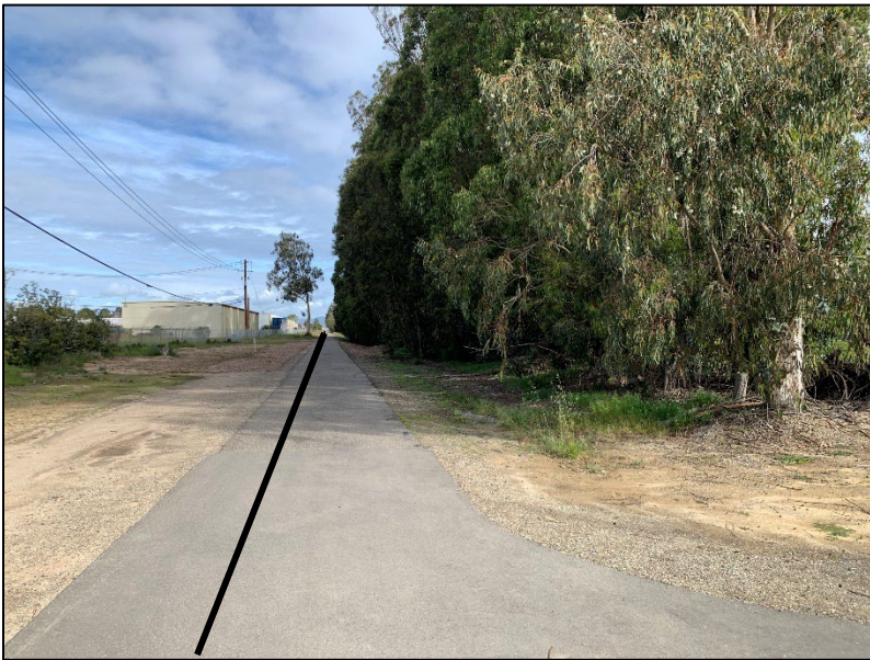
a. Pipeline segment 1 alignment along Santa Maria Valley Railroad Trail
