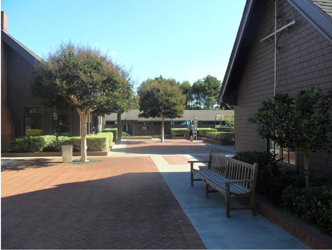
Figure 10a Classroom Building, looking east
