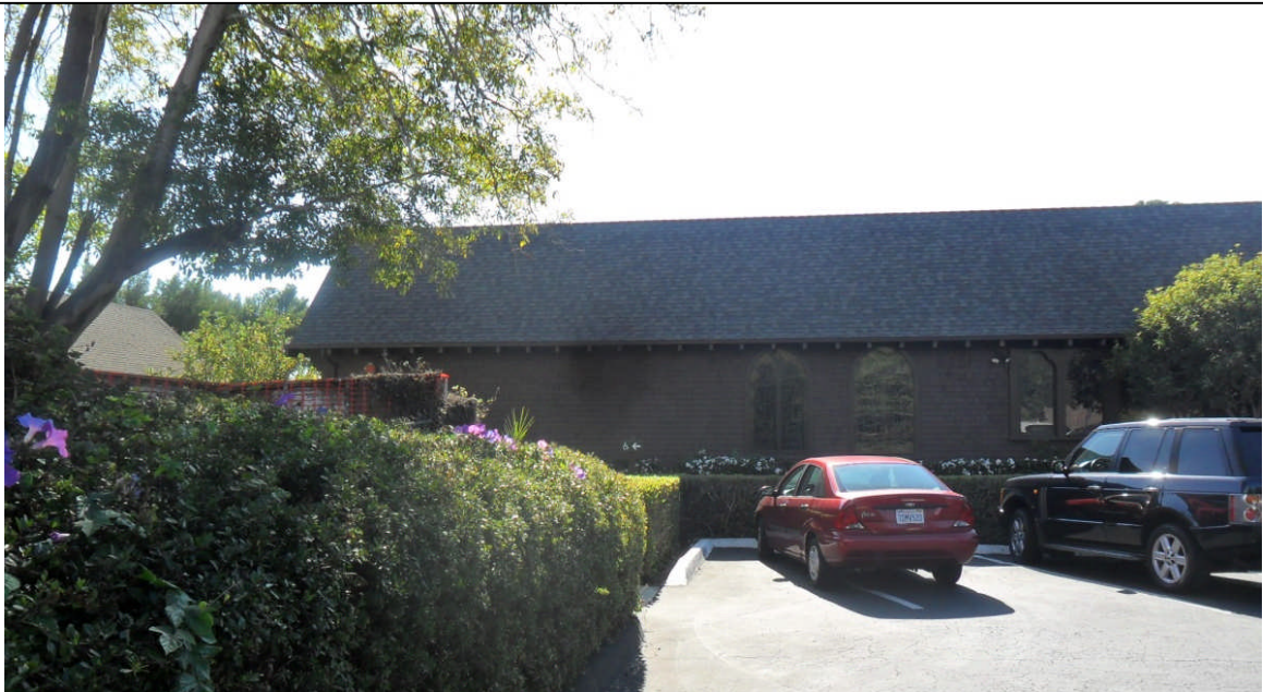
Figure 16 All Saints By-the-Sea Church at 83 Eucalyptus Lane, Montecito North elevation Looking south
