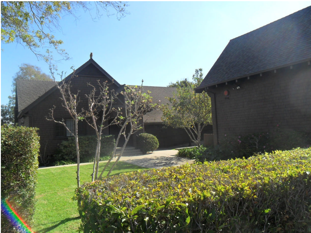
Figure 10b Parish Hall, looking east
