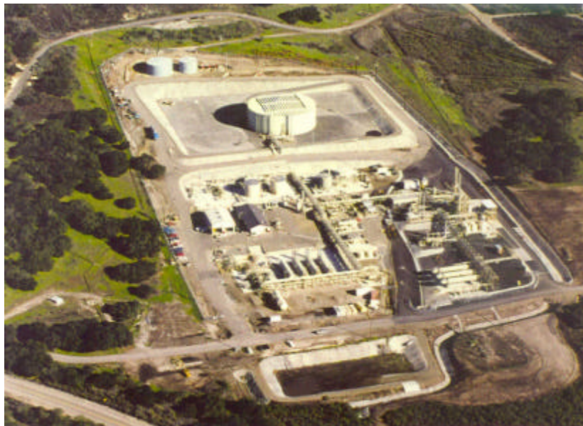
Figure 2 – Lompoc Oil Gas Plant
