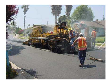
The project consists of in-place recycling of the existing structural section, removing excess material, regrading and compaction of the remaining structural section and paving with Type B asphalt concrete. Approximately 4.51 lane miles of County maintained roadway will be recycled and resurfaced with the construction of this project.
