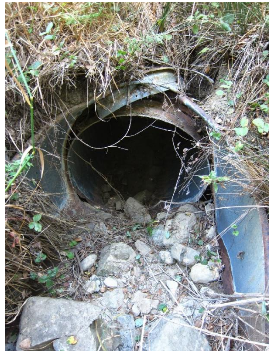
Figure 1: Existing Jalama Rd. Culvert Inlet
