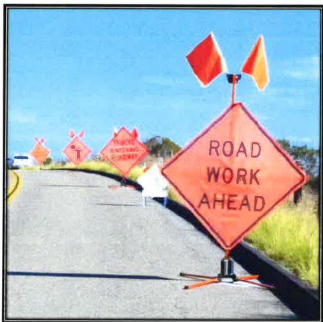
Photo 4: Traffic Controls on Frontage Road (Calle Real)
