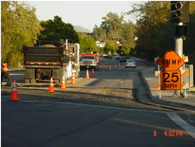
Polyester Concrete Overlay
