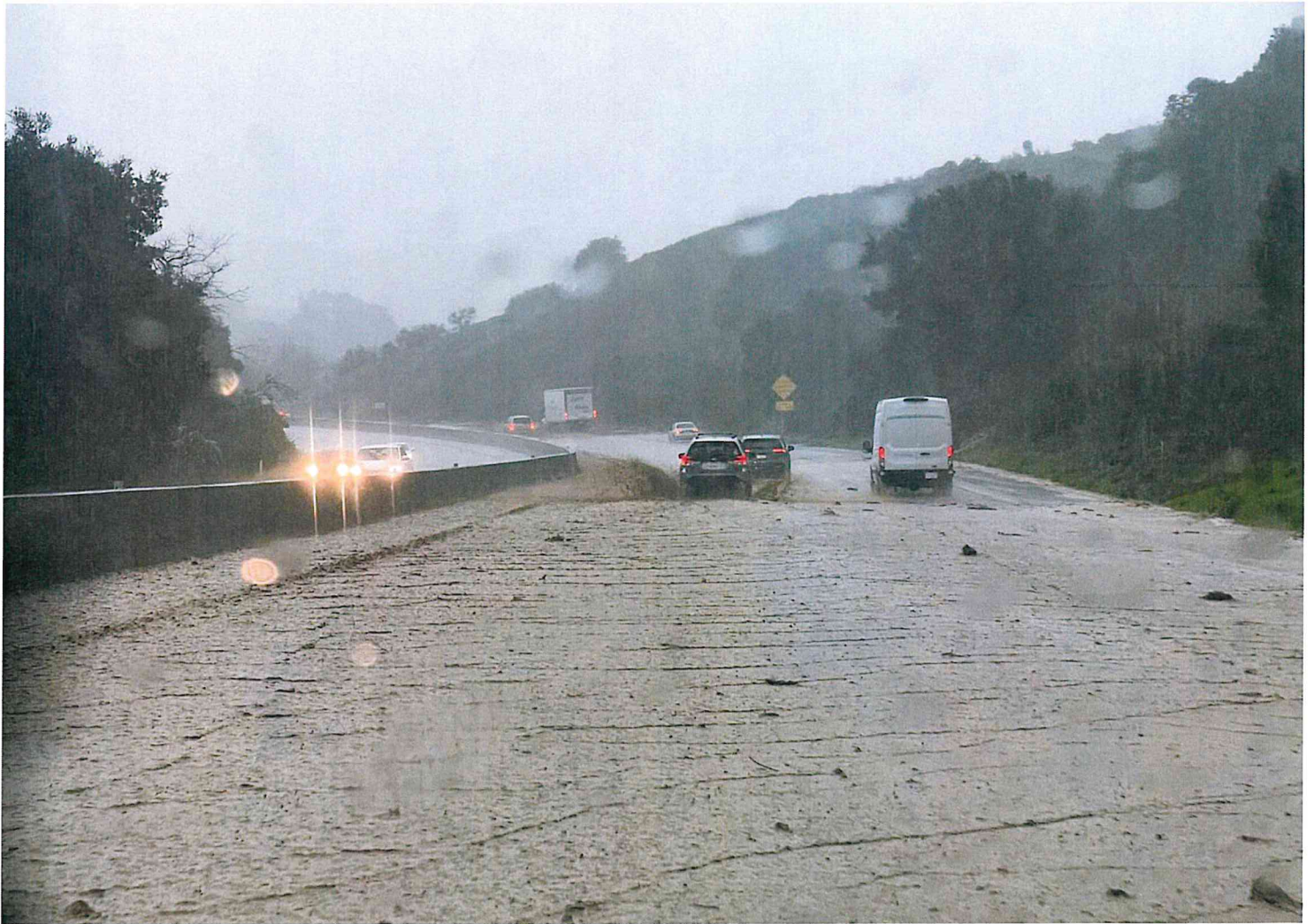
A mudslide covers Highway 101 lanes near the Nojoqui Grade Monday morning. ( Ryan Cullom / Noozhawk photo )
