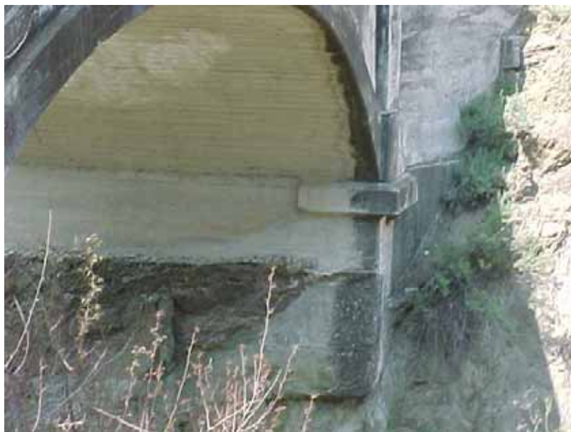
Photo: Existing Bridge 51C-113
