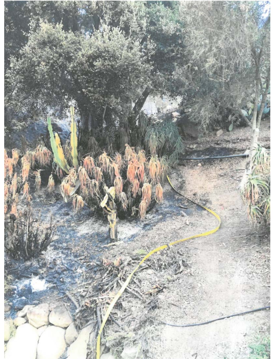
View of fire hose east of accessory building. Fire burned within 10 feet of the building.
