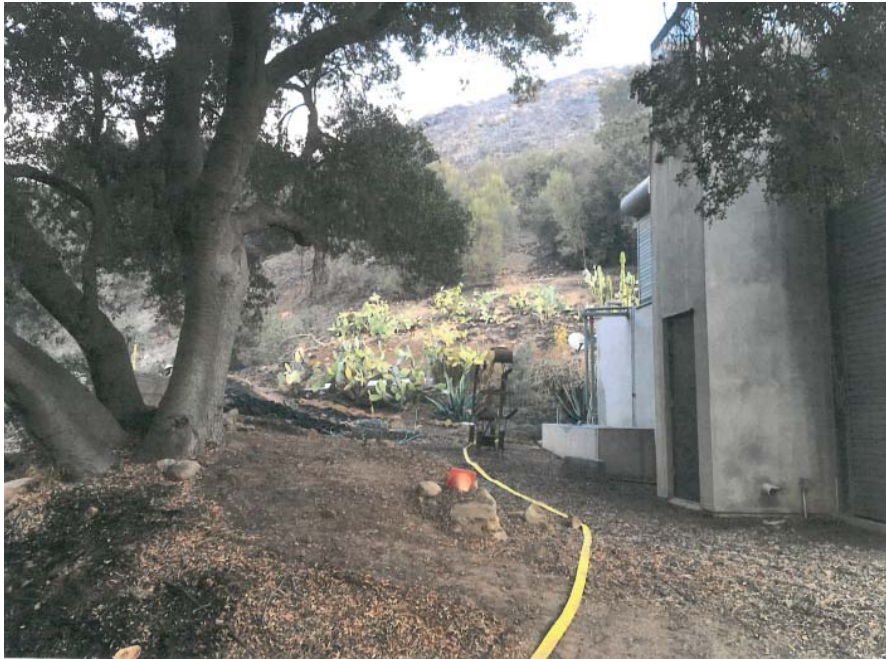
View of fire hose west of accessory building. Fire burned within 10 feet of the building.
