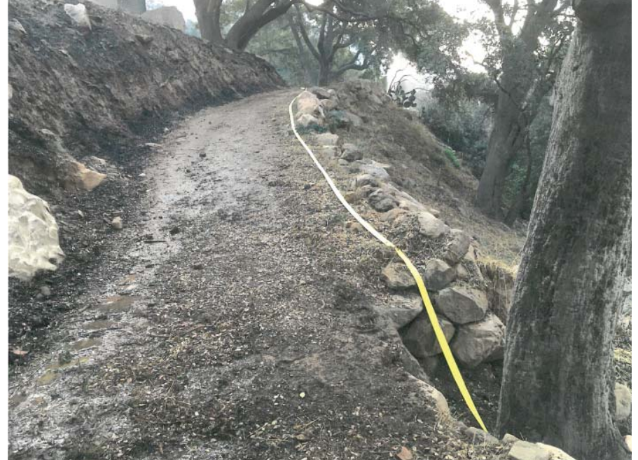
949 Toro Canyon access road 12/14/17. View is south, location is west of accessory building, trail of fire hoses/
