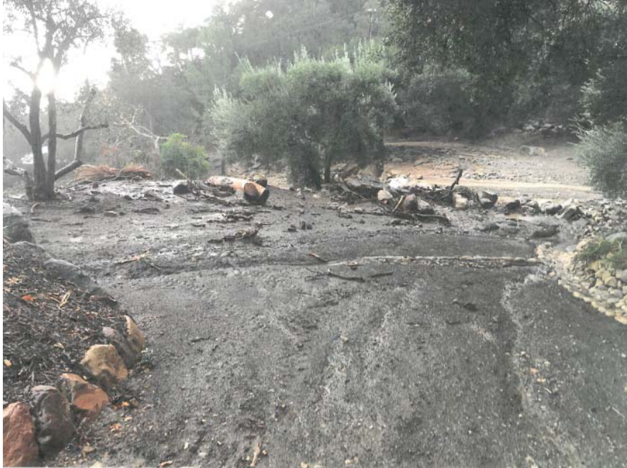
Debris Flow blocking 930/949 Toro Canyon easement and blocking culvert 1/9/18. Supports the need for a second means of egress.
