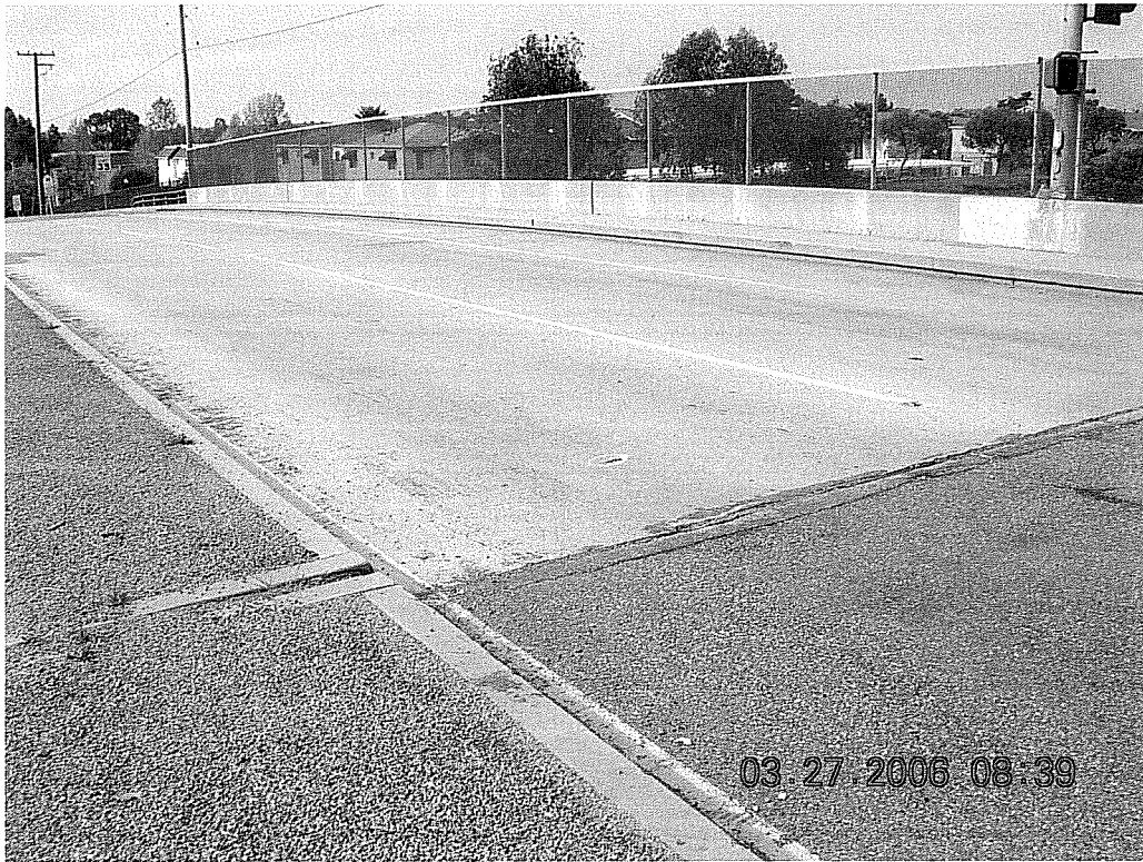
Typical bridge rehabilitation site – Turnpike OH Bridge 51C-154
