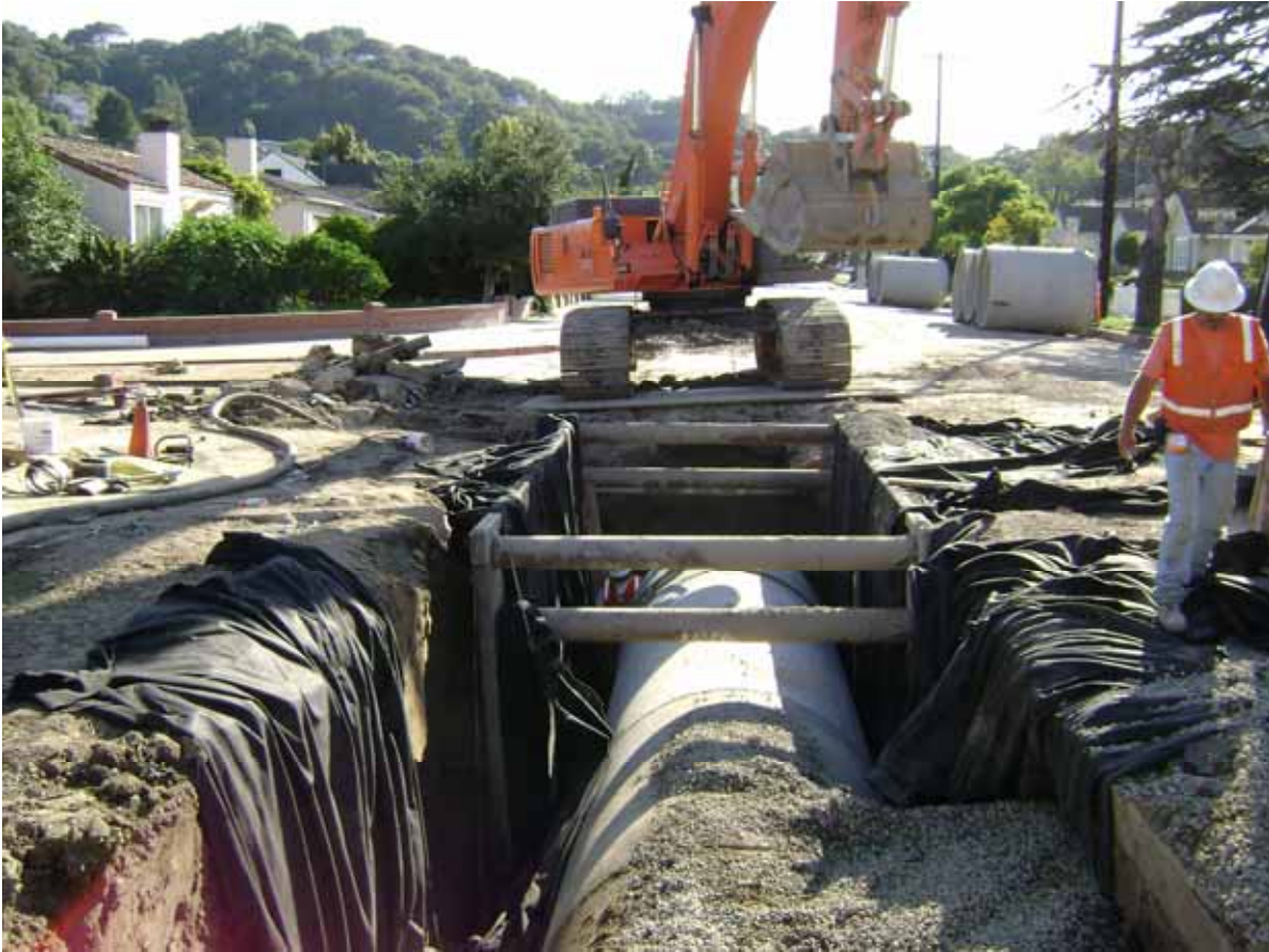
Westside Storm Drain Project Phase III
