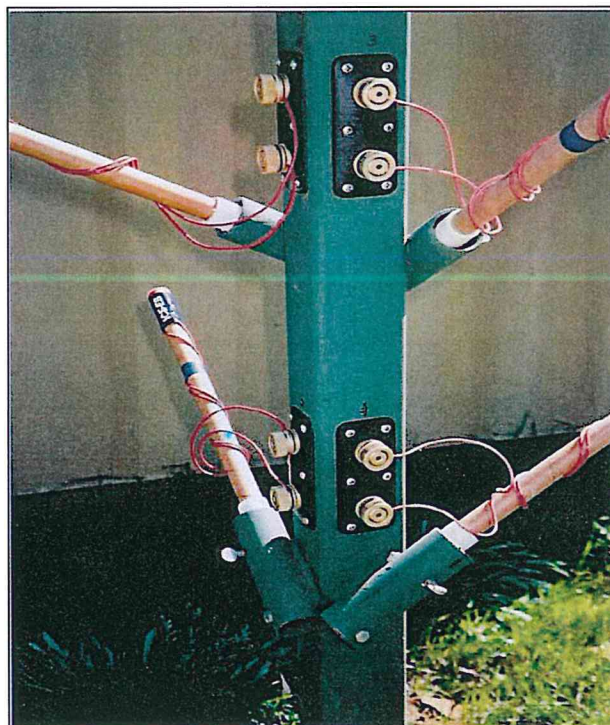
Figure 2.3 Close-up photo of flares
