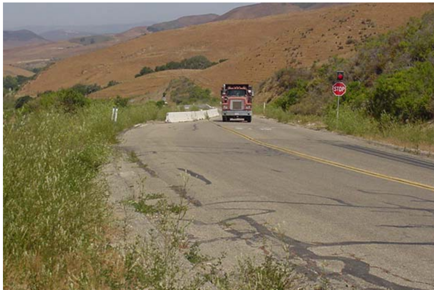
Jalama Road Mile Post 4.4 existing condition, looking north
