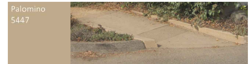
New colored concrete sidewalks.
