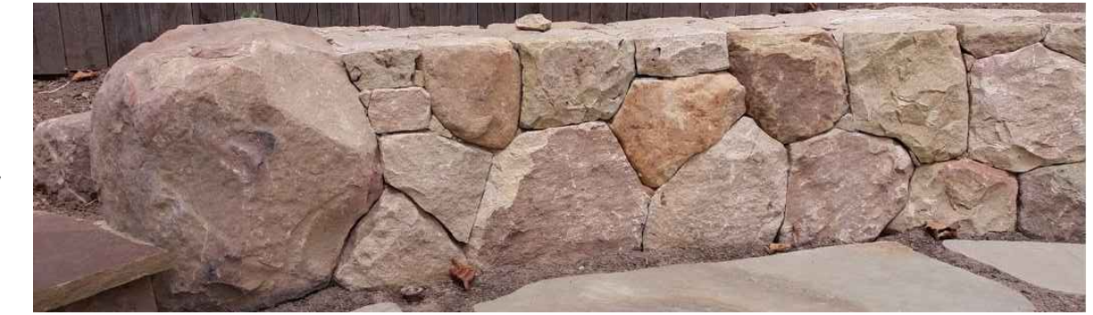
New native sandstone planter wall, 20" high max, with 30" max. high boulders set into wall.
