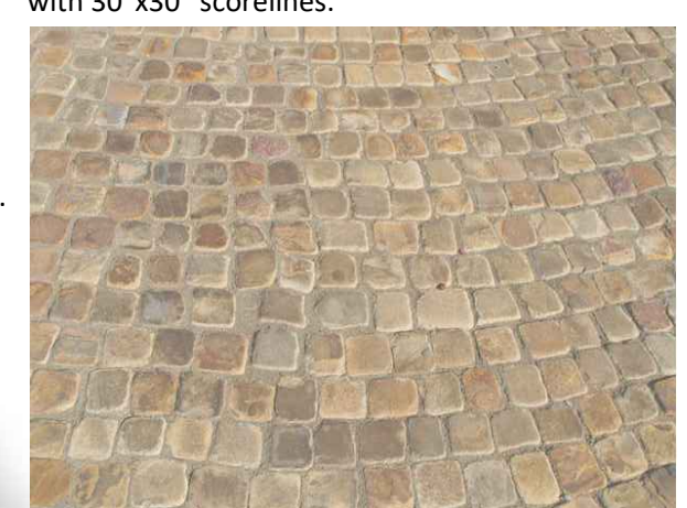
New native sandstone grouted cobble paving.
