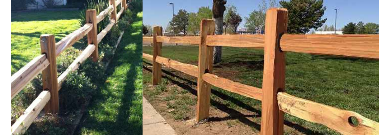
New wood split rail fence. 30" high max. to top rail, 36" high max. to top of posts.
