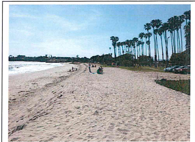
Repairs at Goleta Beach Park have been completed and lie buried beneath the sand (April 2016).
