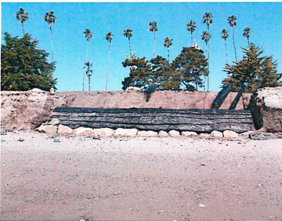
In response to damaging erosion, work crews installed geotextile fabric earth filled cells to protect park facilities in areas that were not already protected by the existing revetment (boulders were temporary and have been removed).
