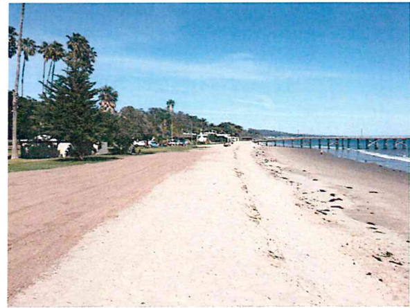
Areas subject to emergency repairs have now been covered with sand by both natural spring time accretion and heavy equipment.
