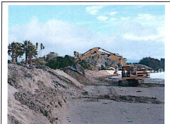
Following completion of the sand berm in December, frequent maintenance involved use of excavators to rebuild the eroding sand berm.
