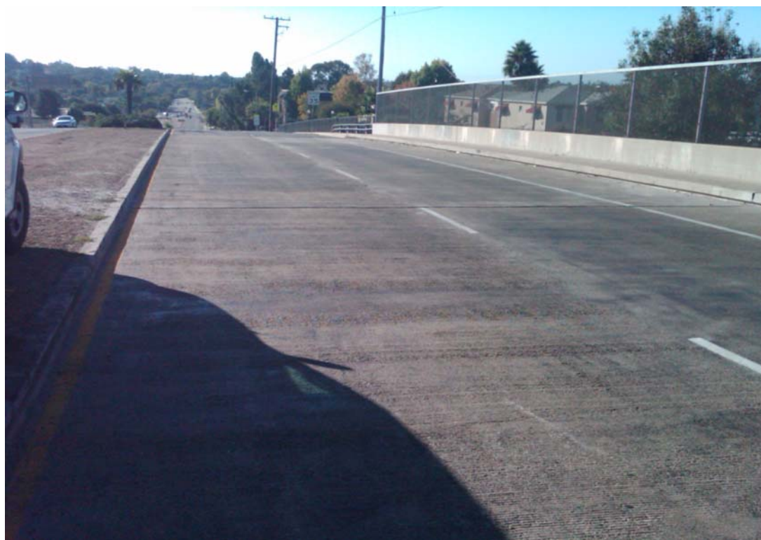
Turnpike OH Bridge 51C-154 – After Bridge Rehabilitation
