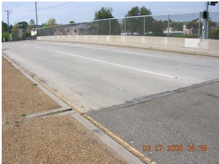
Existing Conditions on Turnpike OH Bridge 51C-154 Prior to Construction
