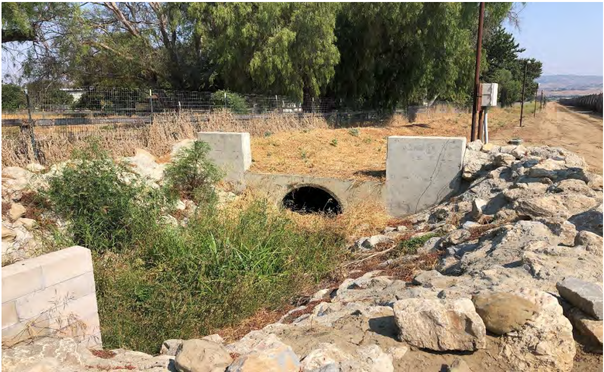
Photograph 10. In-line detention basin upstream of below-ground pipe. (aspect: north; November 1, 2018)
