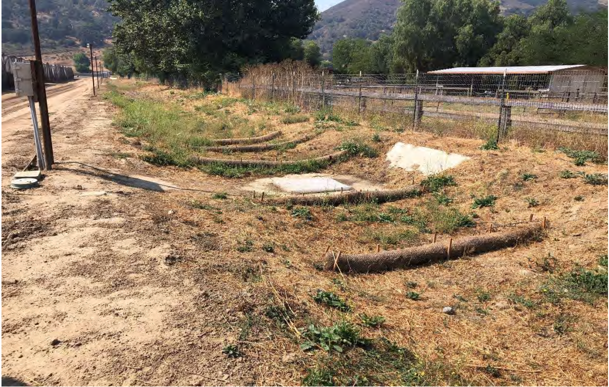
Photograph 9. Detention basin/abandoned agriculture ditch in western portion of the study area. (aspect: south; September 19, 2020)
