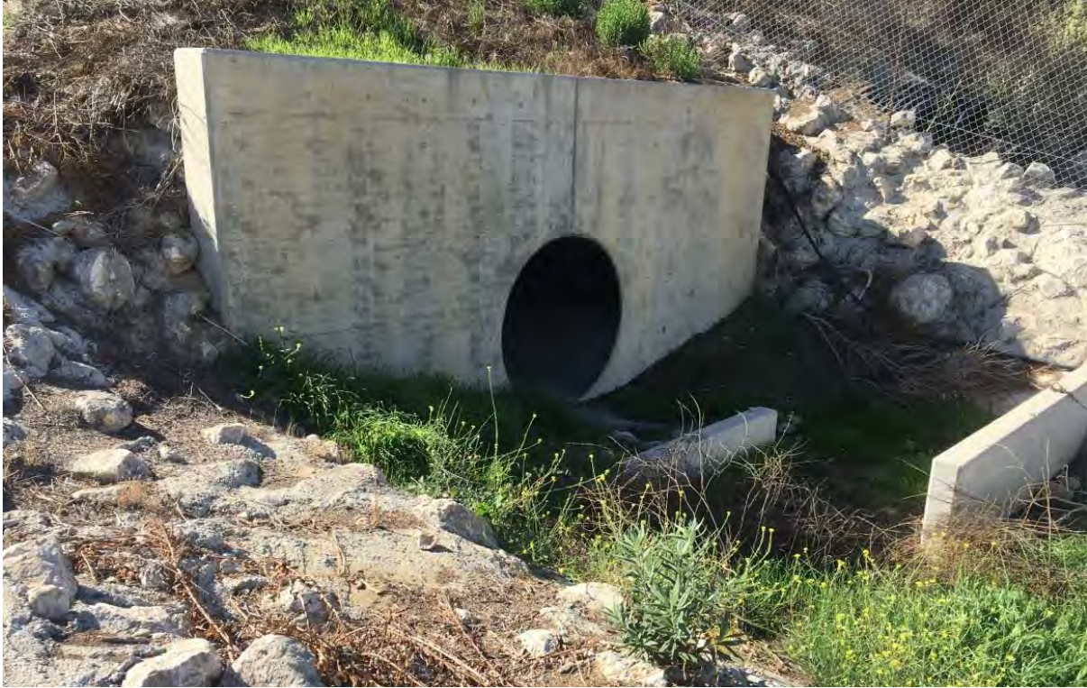
Photograph 5. Downstream terminus of below-ground pipe in western portion of study area draining into in-line detention basin and agriculture ditch, riprap feature visible on left. (aspect: south and upstream; November 1, 2018)
