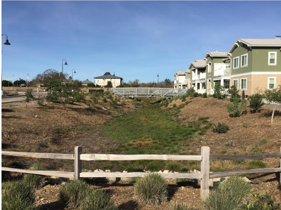
View looking North towards Hwy 246
