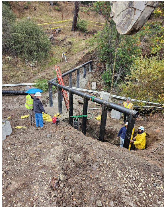
Alamo Pintado Creek Debris Rack Install
