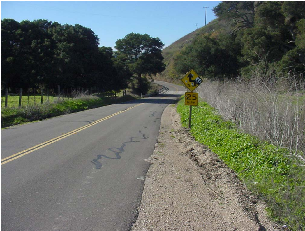
Photo: Existing road alignment heading toward Bridge 51C-016 from HWY 1
