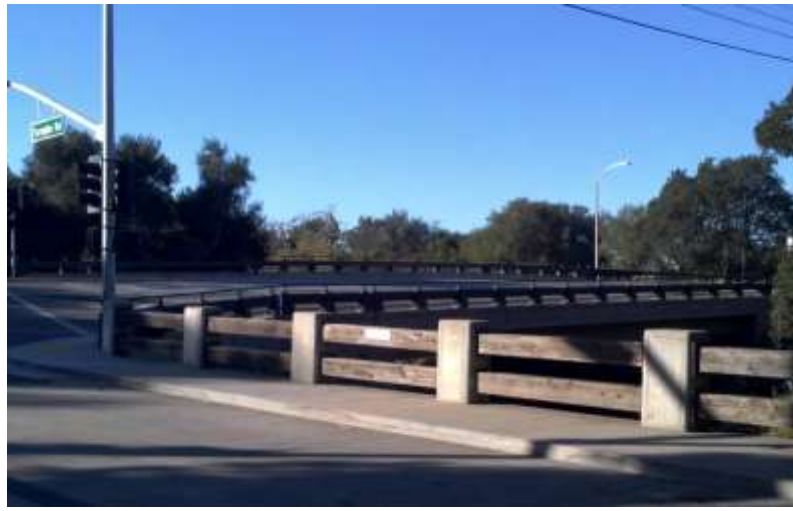
Cathedral Oaks Bridge - Looking From Tucker's Grove Park
