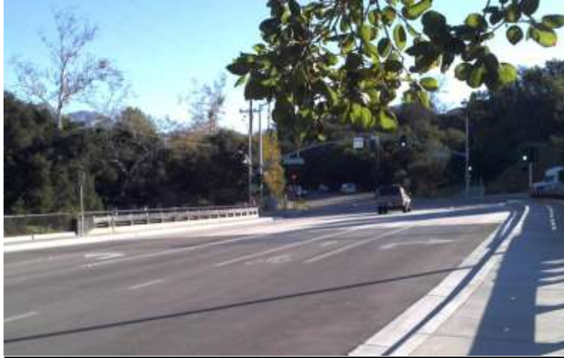
Cathedral Oaks Bridge - Looking East
