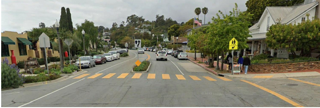
Figure 2: Lillie Avenue, Summerland, CA: at the intersection with Colville Street, looking west
