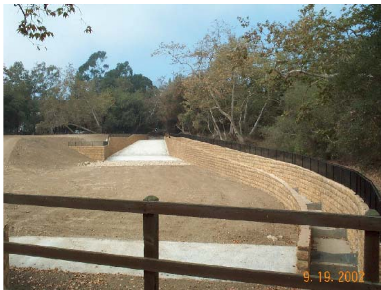
Montecito Creek Debris Basin Completion
