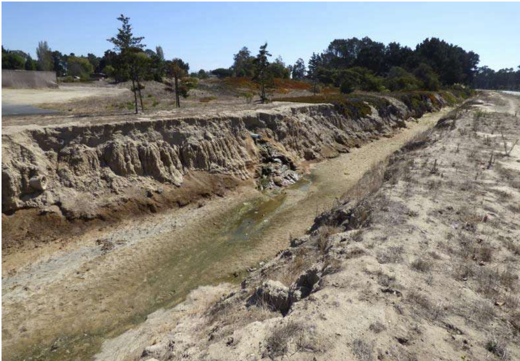
Santa Maria Airport Ditch looking northeast towards Waller Park
