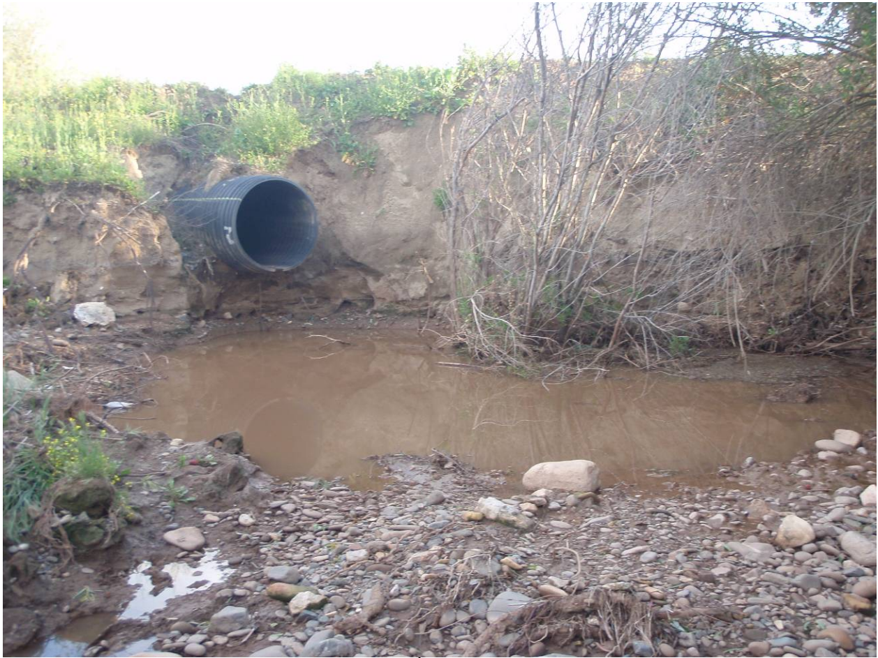
Figure 5: Culvert pool on April 22 nd after considerable drying had occurred.
