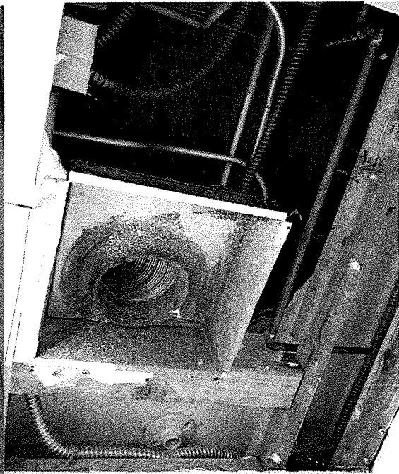
View of the bathroom ceiling in Bldg. 1
