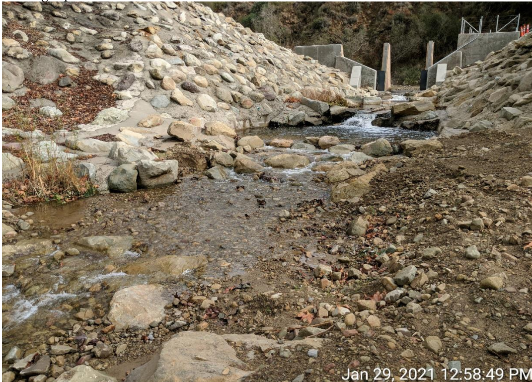
Photograph 6.2-2: Gobernador Creek Debris Basin
