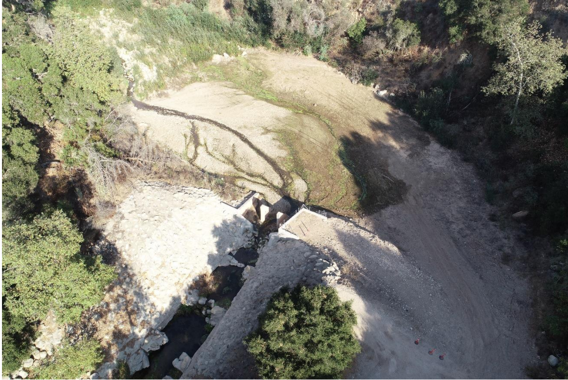
Photograph 6.2-1: Gobernador Creek Debris Basin
