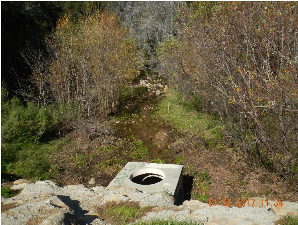
Photograph 5.3-2: Rattlesnake Creek Debris Basin
