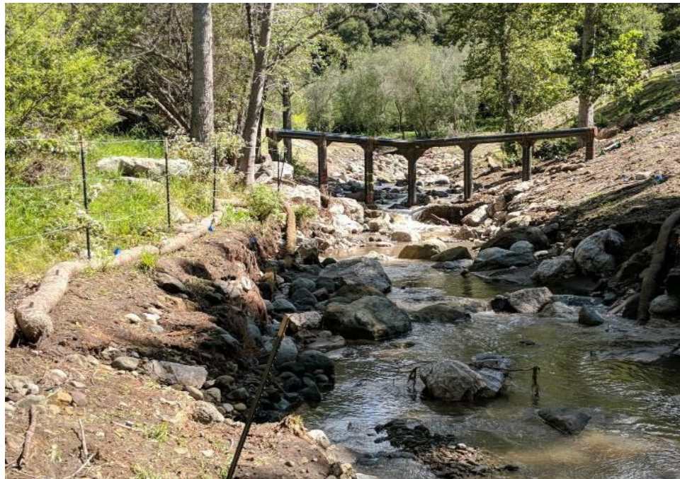
Photograph 4.5-3: Maria Ygnacio Creek Temporary Debris Rack
