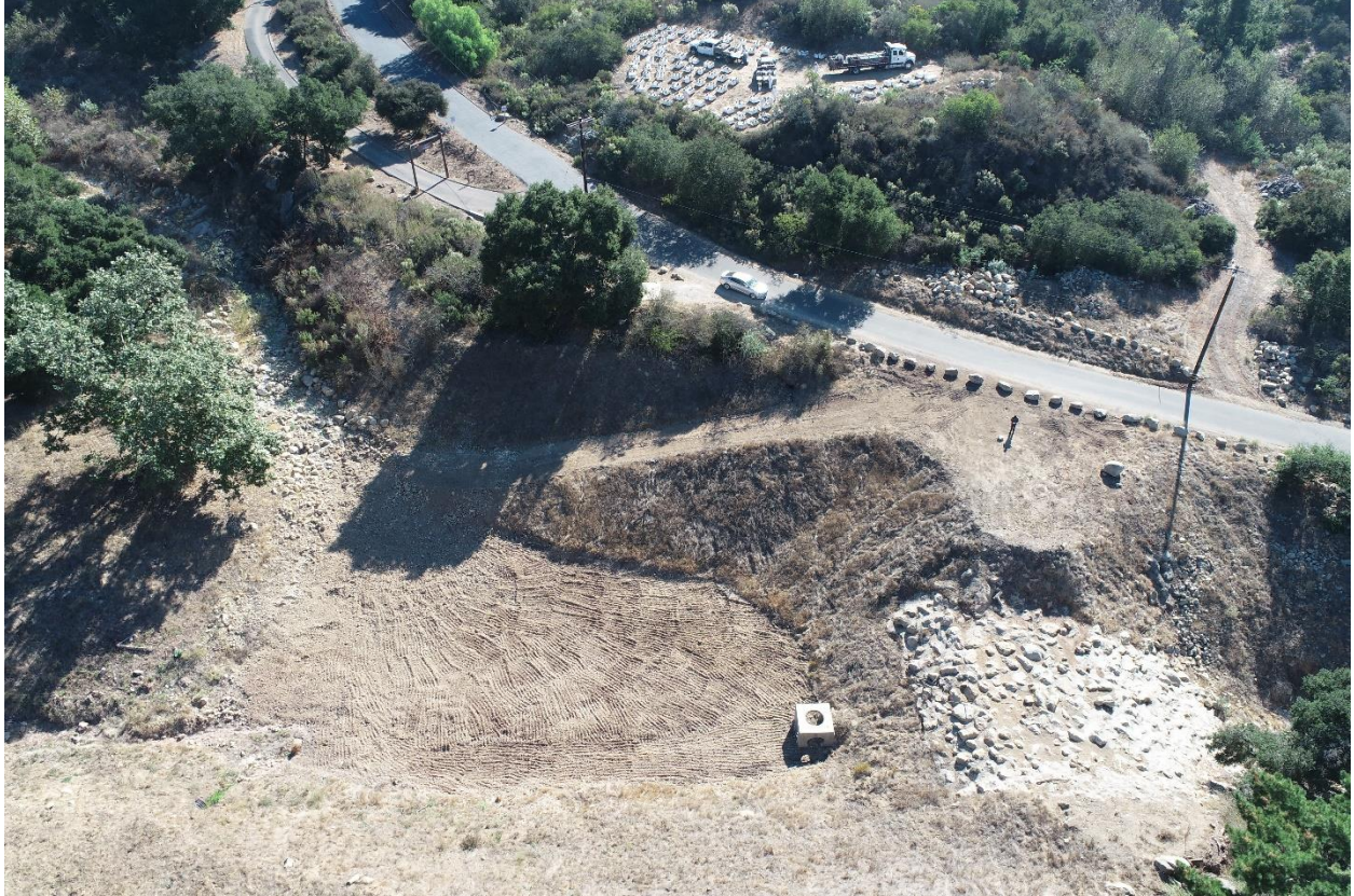
Photograph 5.1-1: Arroyo Paredon Creek Debris Basin
