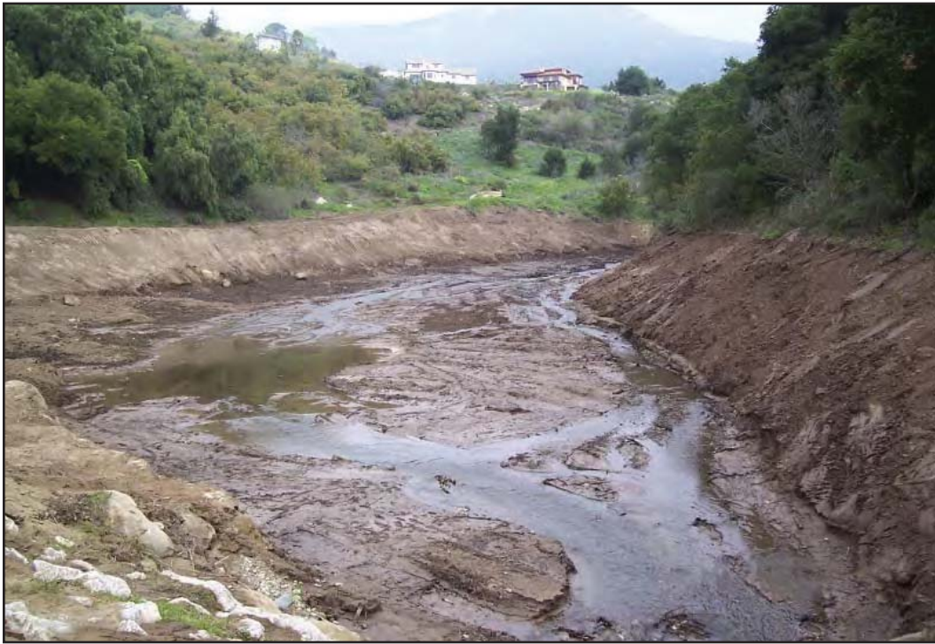
PHOTOGRAPH 2-1 San Roque Creek 2005 Desilting
