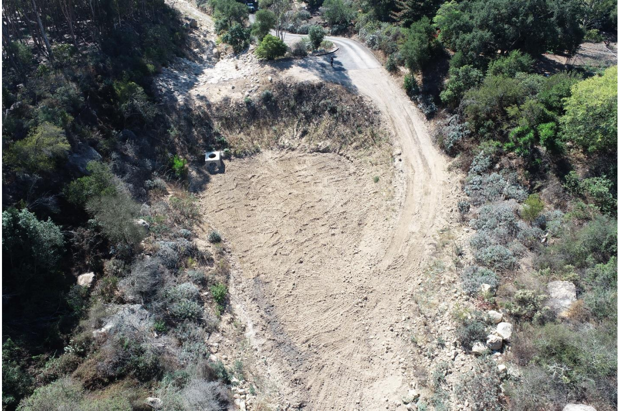
Photograph 6.7-1: Upper West Toro Canyon Creek Debris Basin
