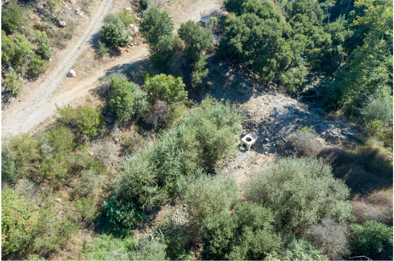
Photograph 5.2-1: Mission Creek Debris Basin
