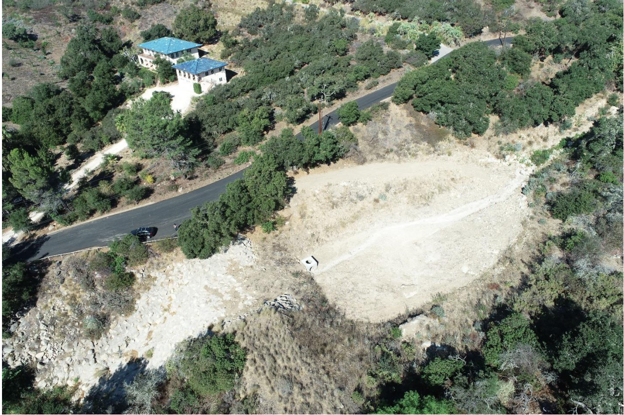
Photograph 6.5-1: East Toro Canyon Creek Debris Basin
