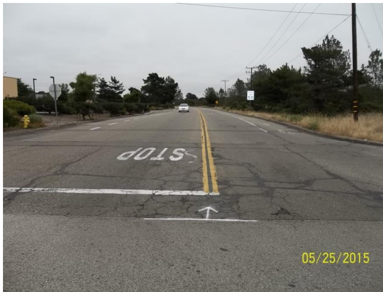
Typical road to be resurfaced (Burton Mesa Blvd.)
