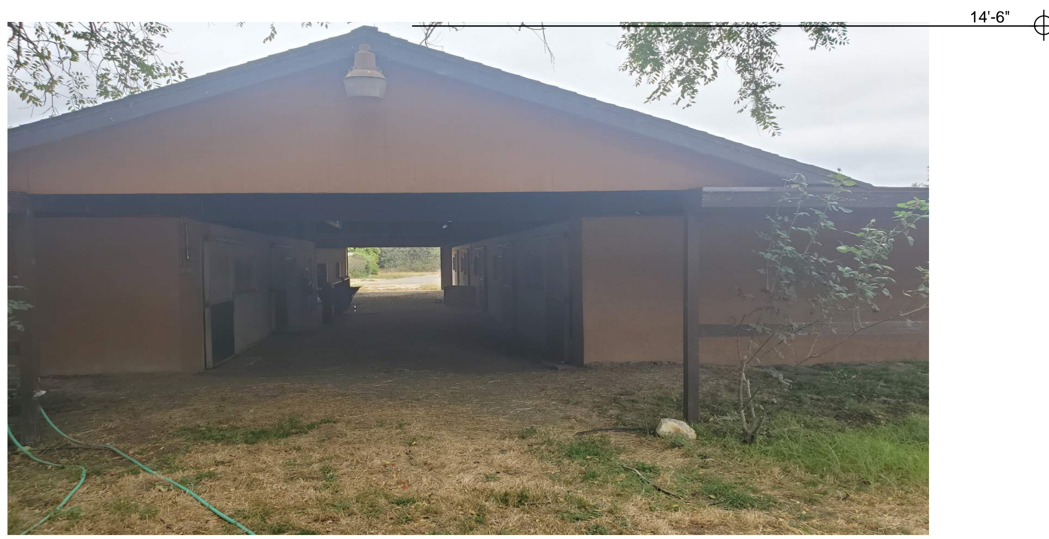
2 A110A NTS EXISTING HAY SHELTER BUILDING SOUTH ELEVATION "NOT UTILIZED FOR CANNABIS OPERATIONS"
