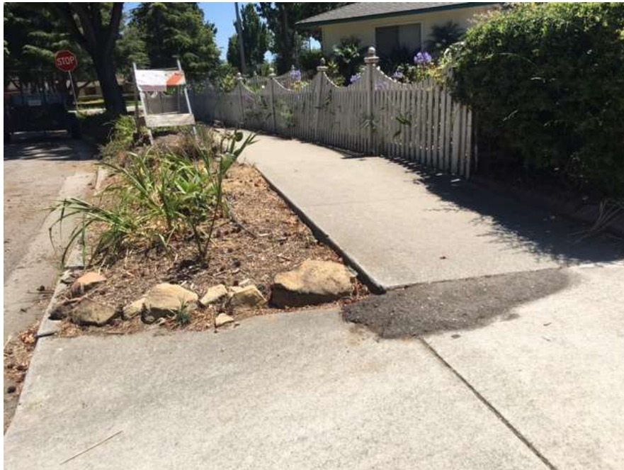
Typical section of sidewalk to be repaired on Santa Paula Avenue
