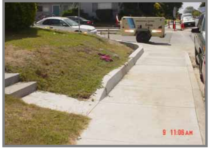
Figure 2: New sidewalk and curb ramp at 850 Cordoba
