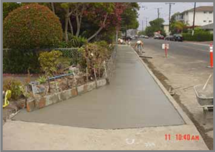
Figure 1: Fresh concrete on Camino Pescadero
