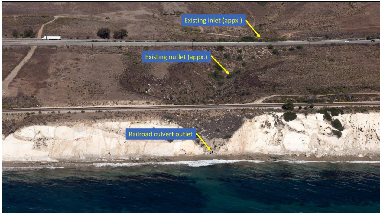
Attachment 3: Aerial photo of the project location
