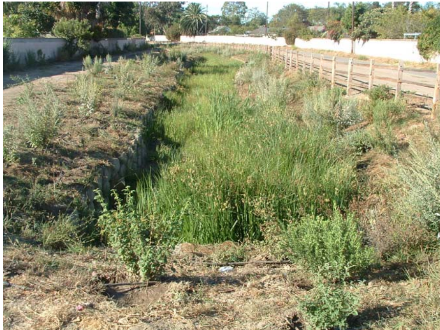
Bioswale establishment (August 2003)
