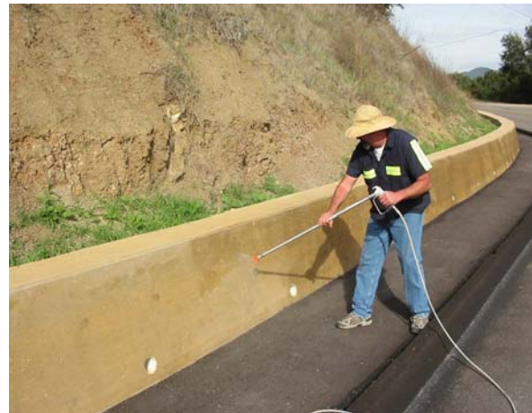
Bluff Colored Retaining Wall and Berm
