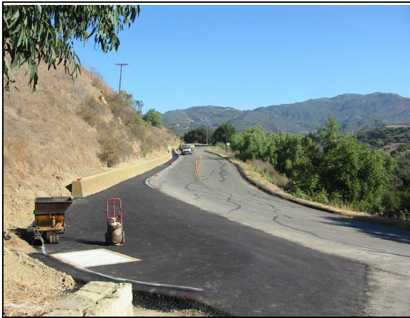
San Marcos Road at MP 0.7
