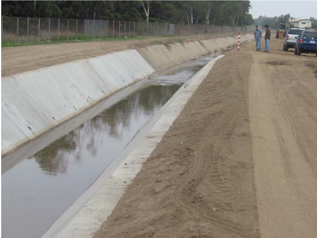
Bradley Channel Repair Project Completion
