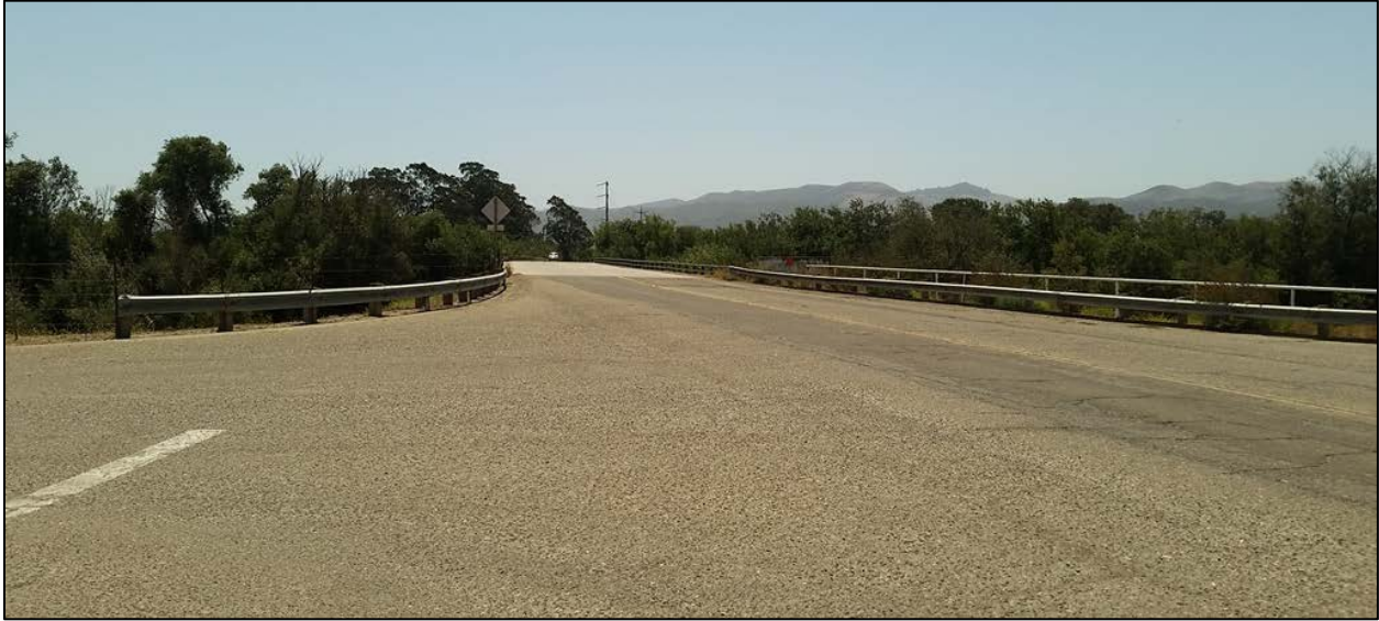
(a) Southward View of Bridge Approach from Santa
