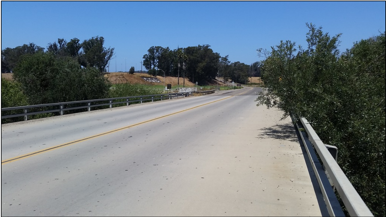
(b) Northward View from existing Floradale Avenue Bridge
