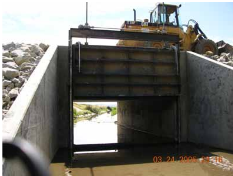
West Green Canyon Storm Drain Project
