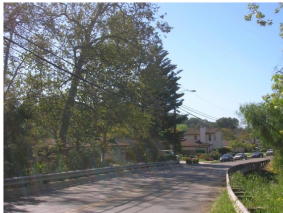
San Marcos Road Bridge No. 51C-002, looking South
