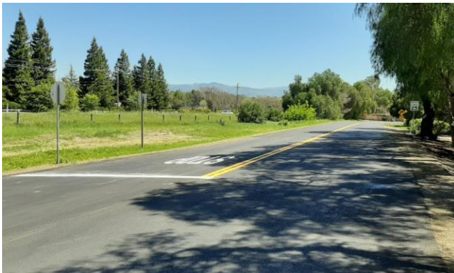
Project No. 820758 – Steele Street Rehab
