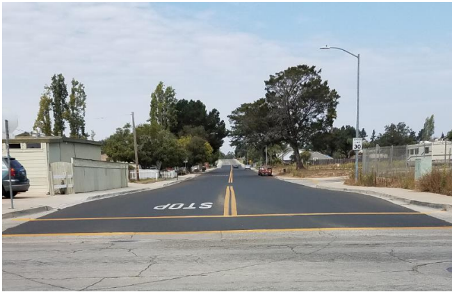
Project No. 820683 – Preventive Maintenance
