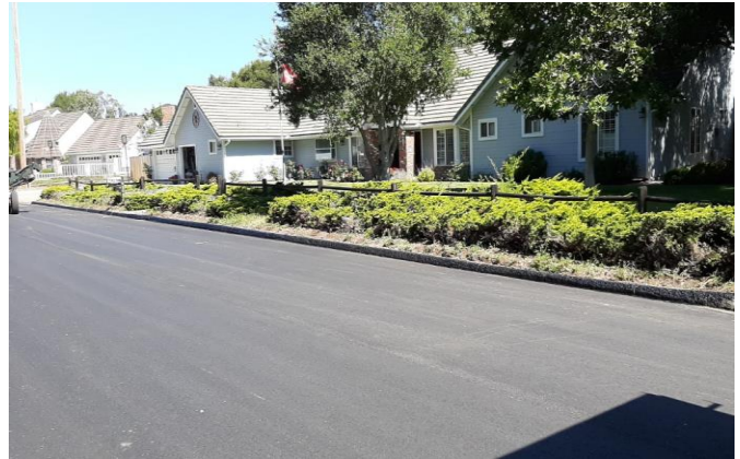
Project No. 820757 – Pellham Drive Rehab
