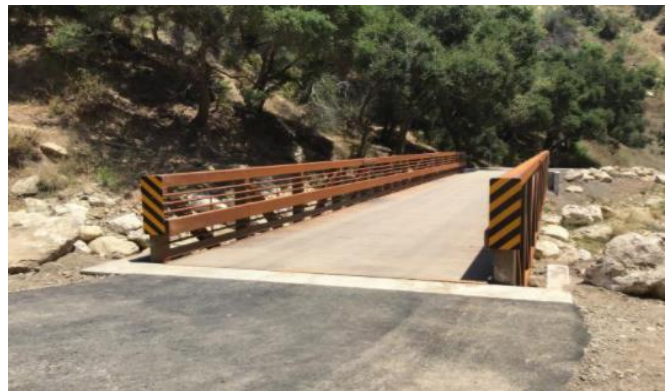
Project No. 862420 – E. Mountain Dr. Temp Bridge
