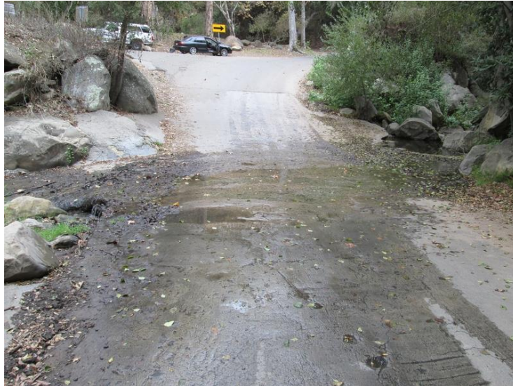
Photograph 1. Low Water Crossing Pre-TFDFI, September 2016 (view west)
