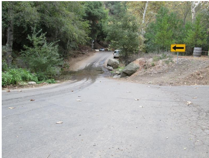
Photograph 2. Low Water Crossing Pre-TFDFI, September 2016 (view east)
