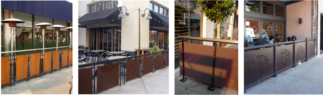
Figure 3.6 - Metal railings with solid panel inserts
