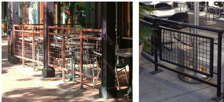
Figure 3.8 - Metal railings with wire mesh panels
