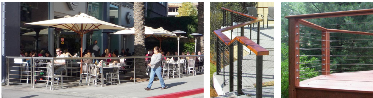
Figure 3.7 - Metal or wood railings with horizontal cables
