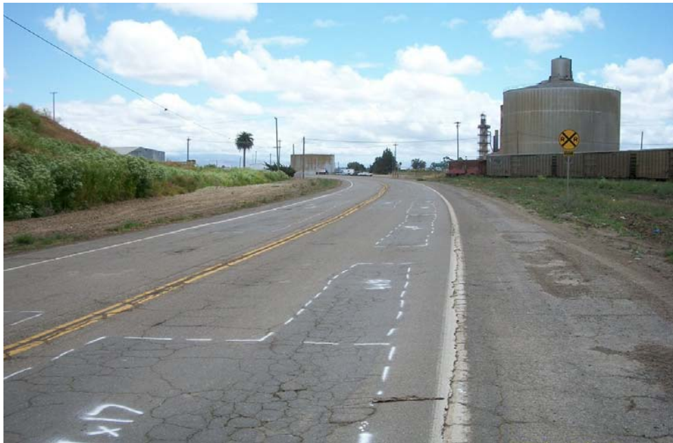
Betteravia Rd, typical to be rehabilitated
