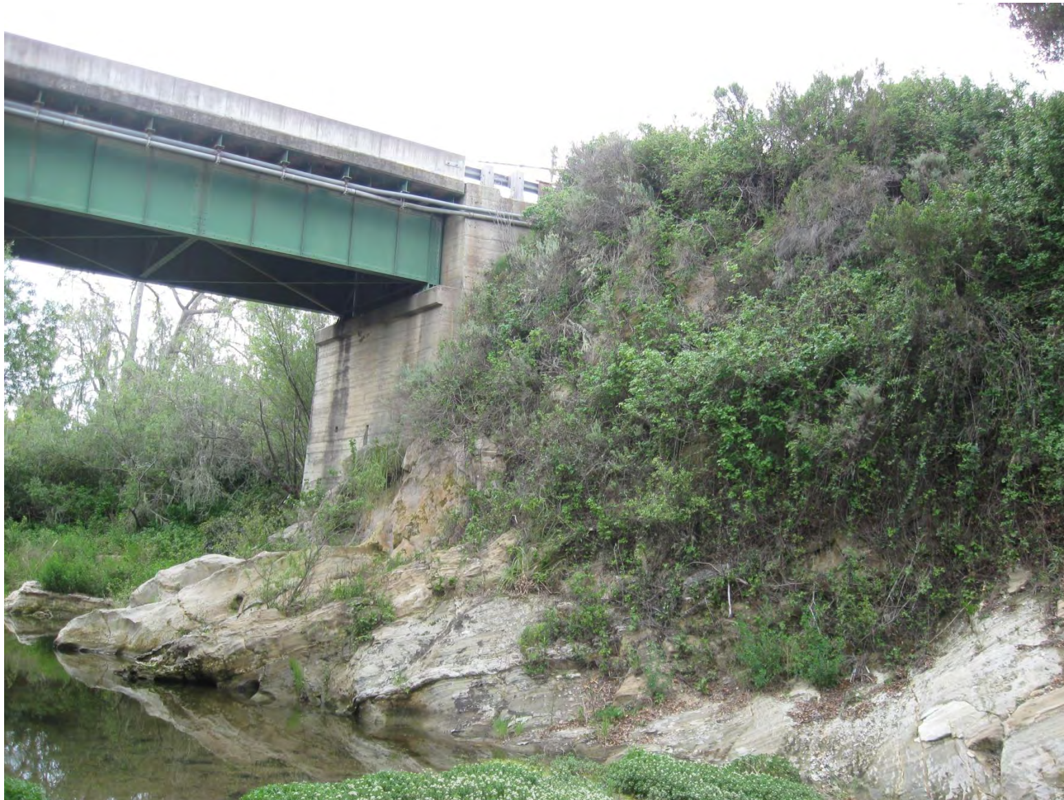
Photo 11 Looking at northwest slope
