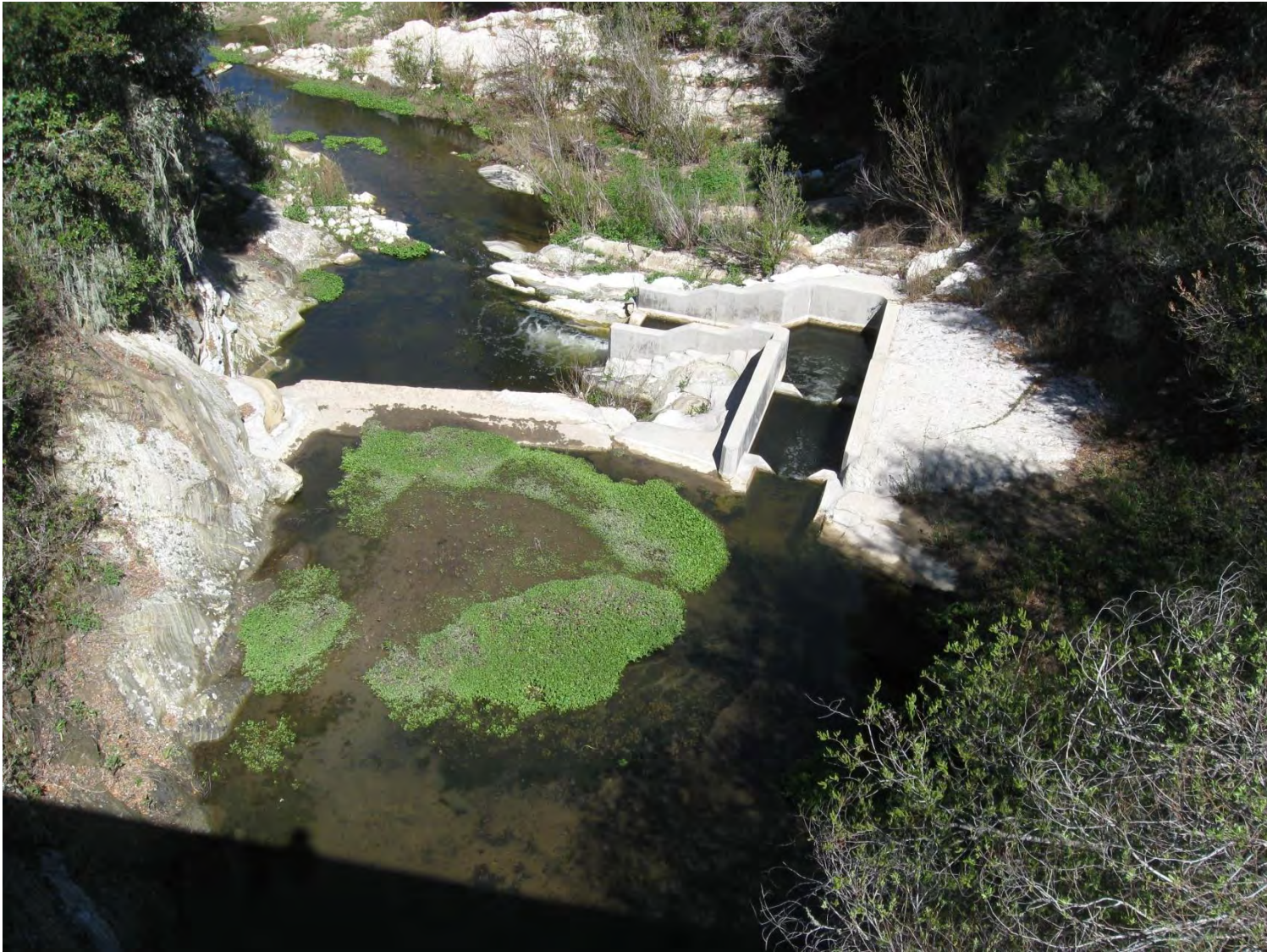
Photo 8. Salsipuedes Creek looking upstream from the Jalama Road Bridge
