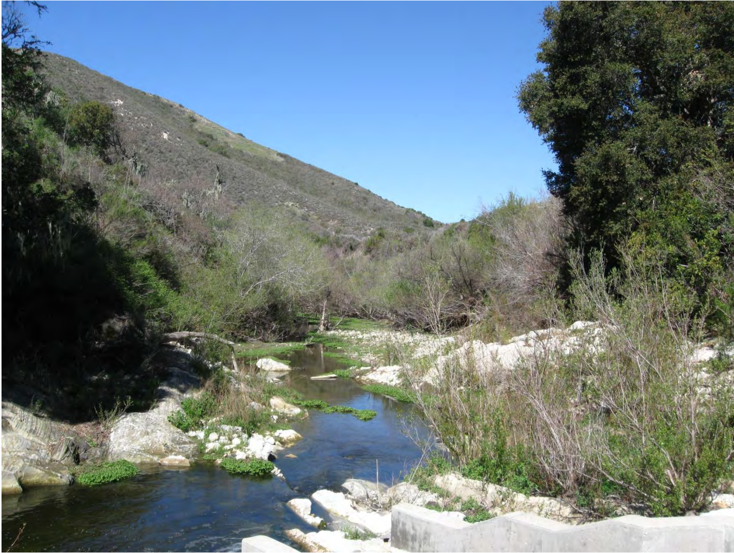
Photo 7..Salsipuedes Creek looking at Fish Ladder and Pools on downstream side of Jalama Road Bridge
