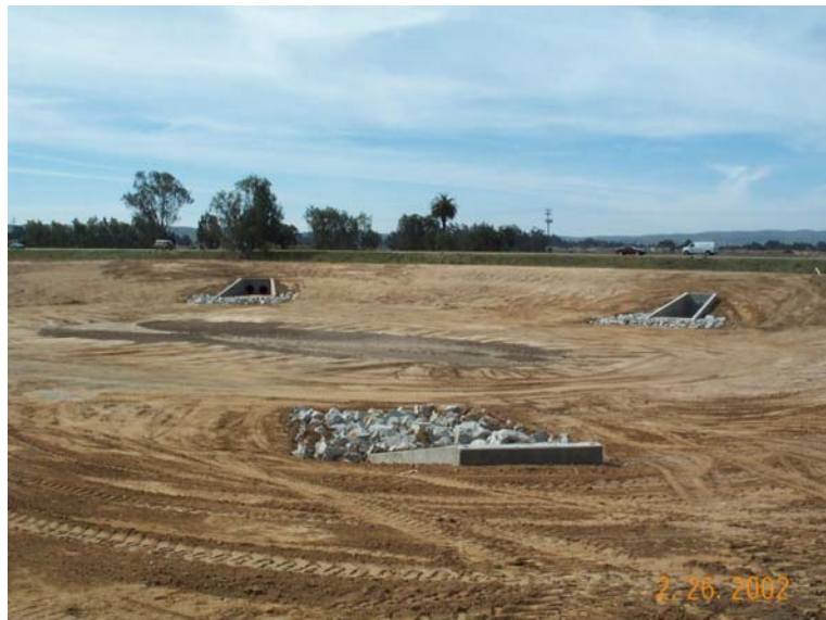
Prell Basin Completion
