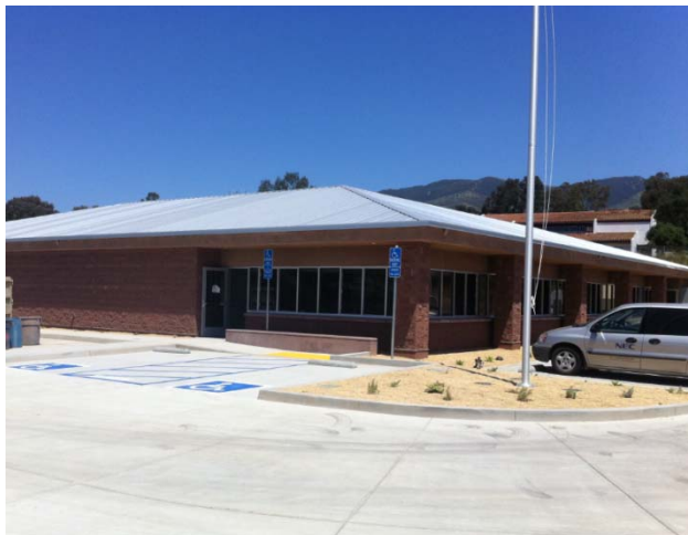
Emergency Operations Center $5.4 m
