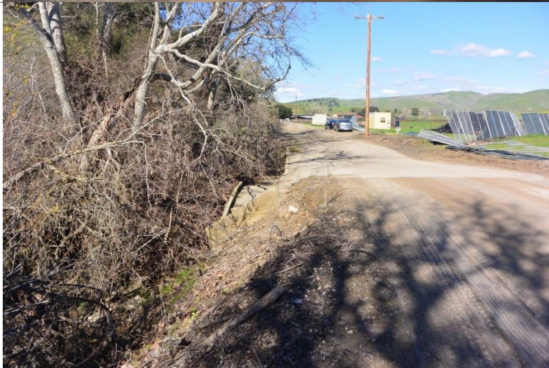
Photo 15. Crossing #4: Concrete-paved, low-water "summer crossing" located along gravel access road, southwest of 16.53-acre cultivation area. (photo taken 2/7/2019)
