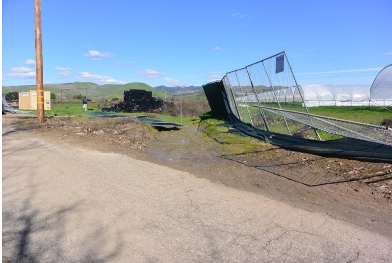
Photo 16. Ephemeral watercourse (Class III) west of 2018 cultivation site. Reaches concrete summer crossing. (photo taken 2/7/2019)
