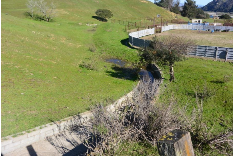
Photo 43. Man-made drainage system (Class IV watercourse) near proposed 2.55-acre cannabis premises area. (photo taken 2/7/2019)
