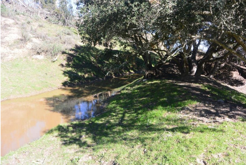
Photo 34. Man-made pond, part of man-made drainage system, located adjacent to (north of) 1.79-acre future cultivation area. Potentially created for groundwater recharge. (photo taken 2/7/2019)
