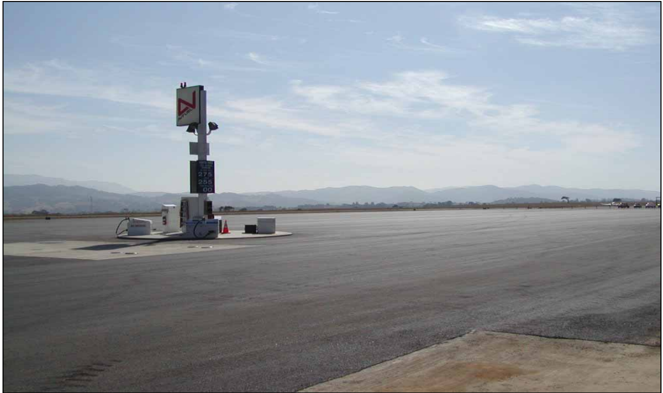
Photo: Completed SY Airport Apron Rehabilitation
